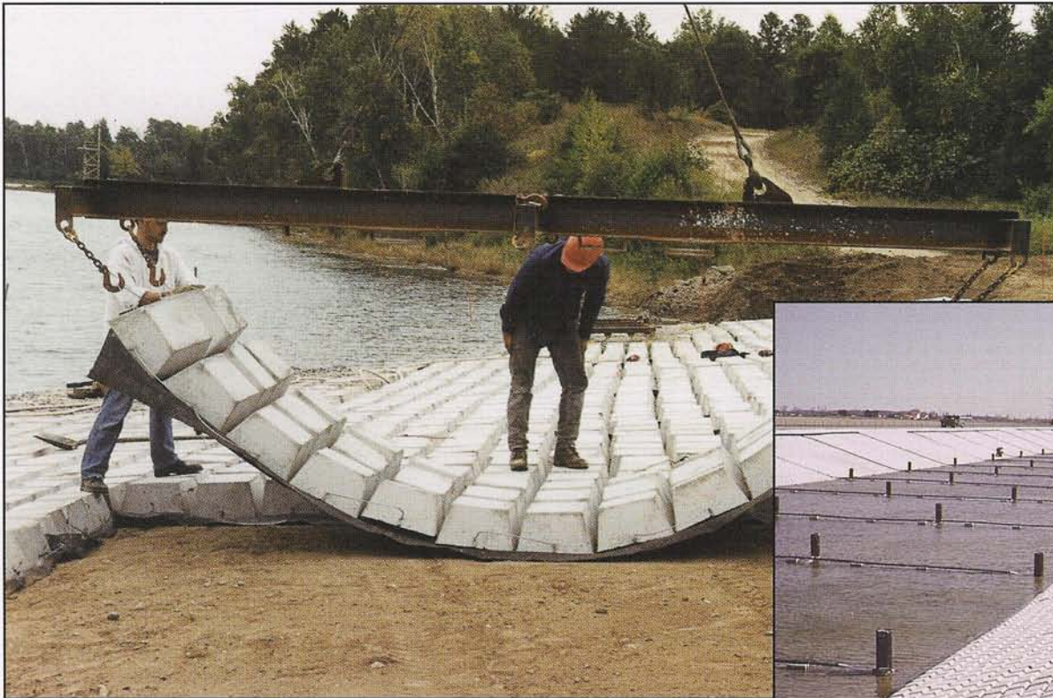
Articulating Concrete Block
