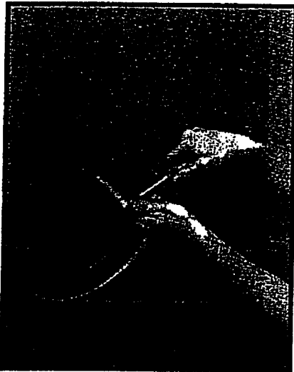
Install Kor-N-Seal I - Wedge Korband With Socket Wrench & Torque Limiter
